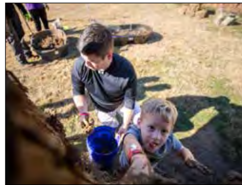
Photos by Christian Toews Ezekiel Fincher presses a mixture of clay, water, and hay/grass onto a traditional Choctaw home to insulate it from the coming winter weather.
