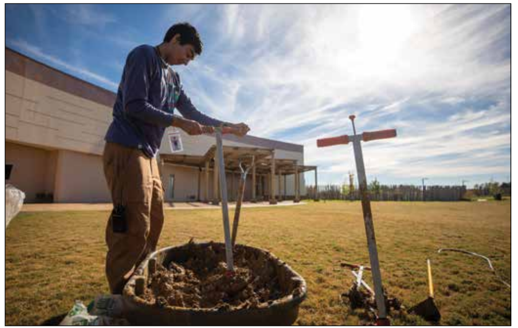
Kaleb Standridge uses tools to help mix the clay to the proper consistency, allowing it to stick to the outside of the traditional shelter.
