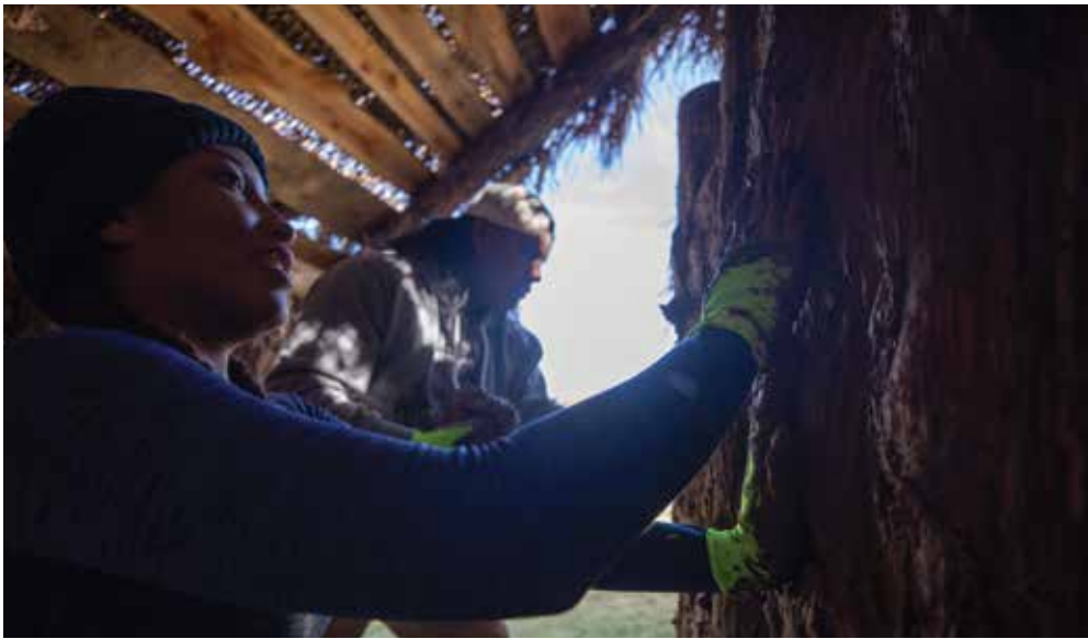
Aliiah Myers and Demetrius Williams spread clay near the entrance of the traditional shelter.
